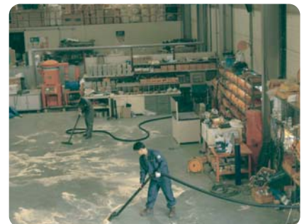
Factory cleaning system
